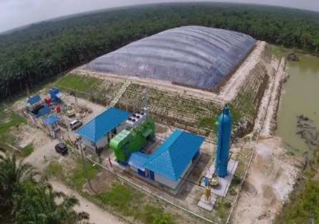
Commissioning PLT Biogas Desa
