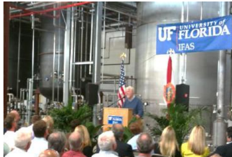
Customer Installation University of Florida
