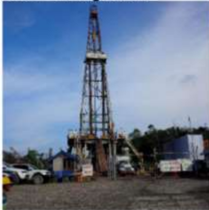
SIL 1n – Drilling SIL1n-2
